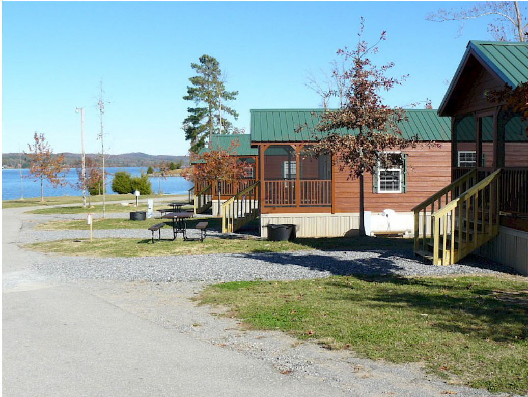
Cabins purchased and installed by RRM at Lake Guntersville SP
